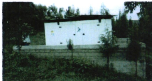
Proposed Construction of 2 No. Generator Houses
