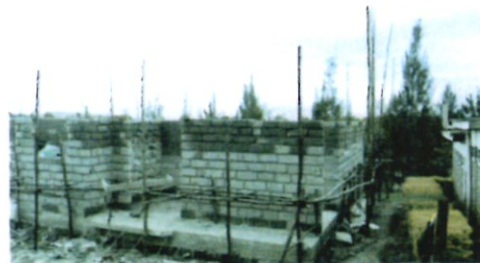
Construction of 2NO. Ablution Blocks
