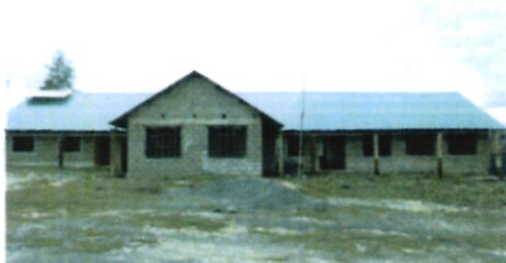
Construction of Research Collaboration, International and Training Centre/Units
