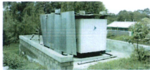
Proposed Construction of 2 No. Generator Houses
