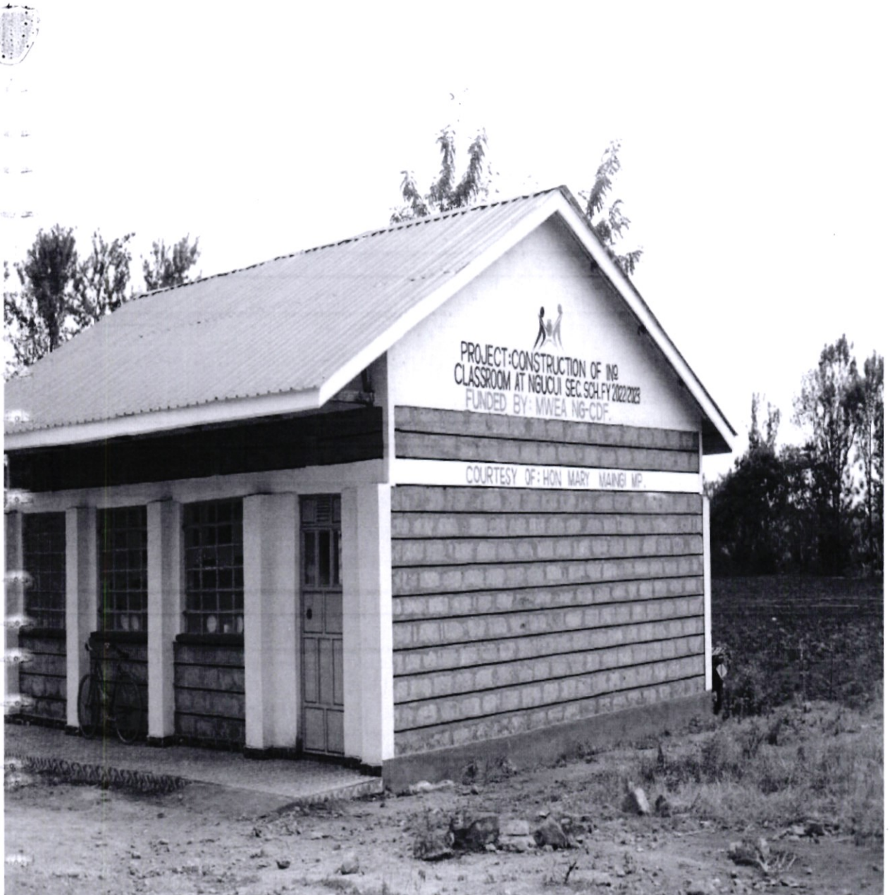
A standard classroom at Ngucui secondary school
