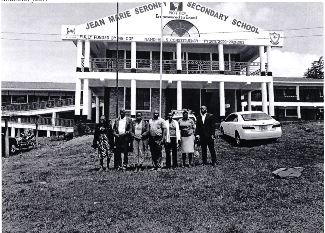
Jean Marie Seroney Secondary School-Construction of Tuition and Administration Block
