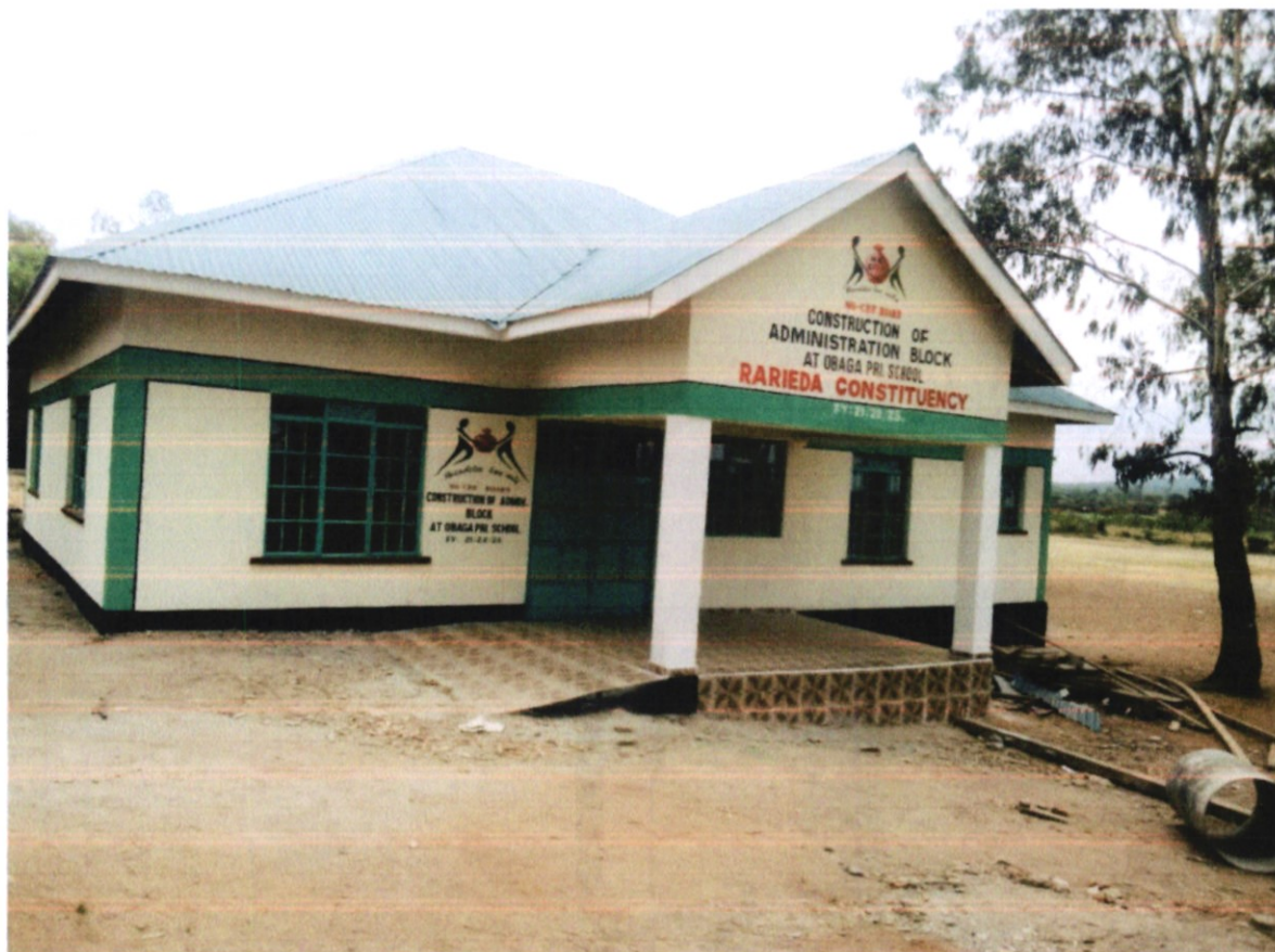
Figure 2: Construction of Admin Block at Obaga Primary School
