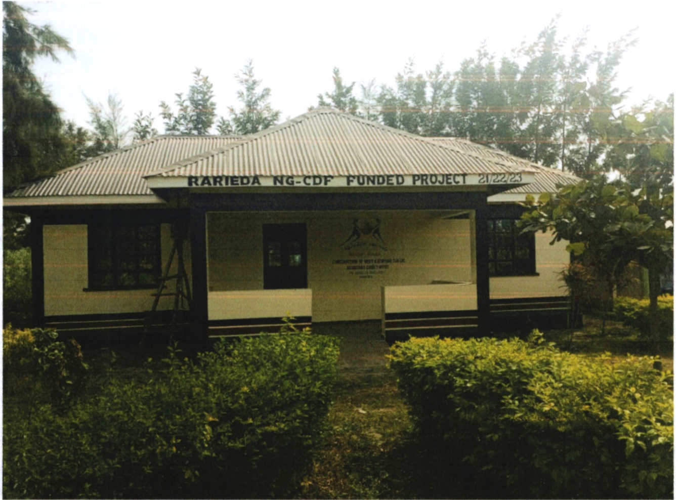
Figure 14: Completion of West Katwenga Assistant Chiefs Office
