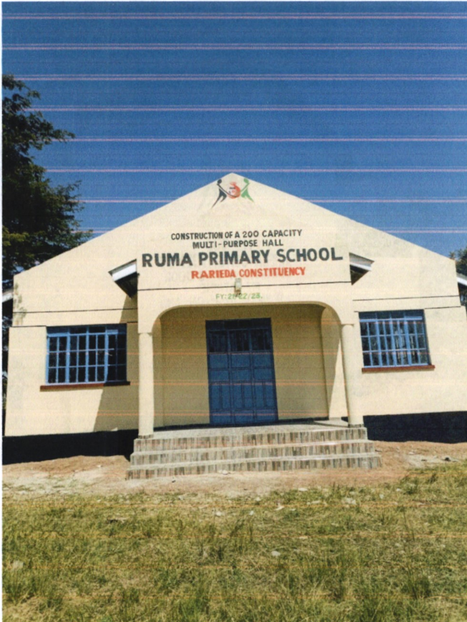
Figure 11: Construction of a 200 capacity Multi-Purpose Hall At Ruma Primary School
