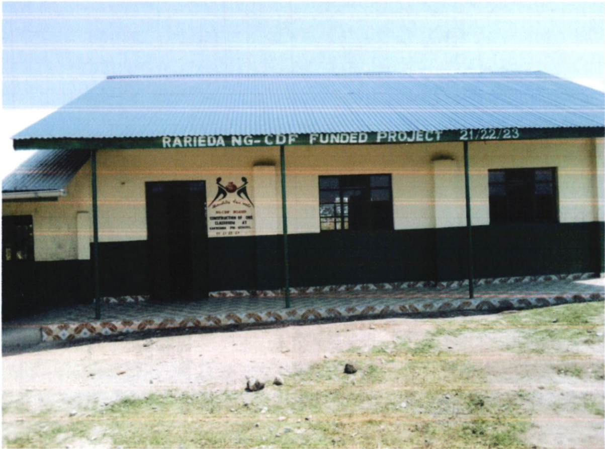
Figure 6: Construction 1No. classroom at Kakremba Primary School
