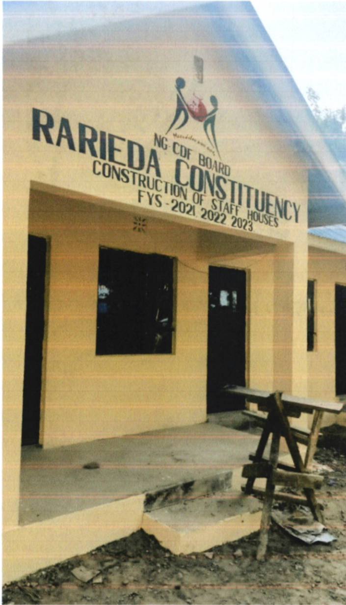
Figure 3: Construction of staff Houses at Owimbi Administration Police Camp(Central Uyoma)
