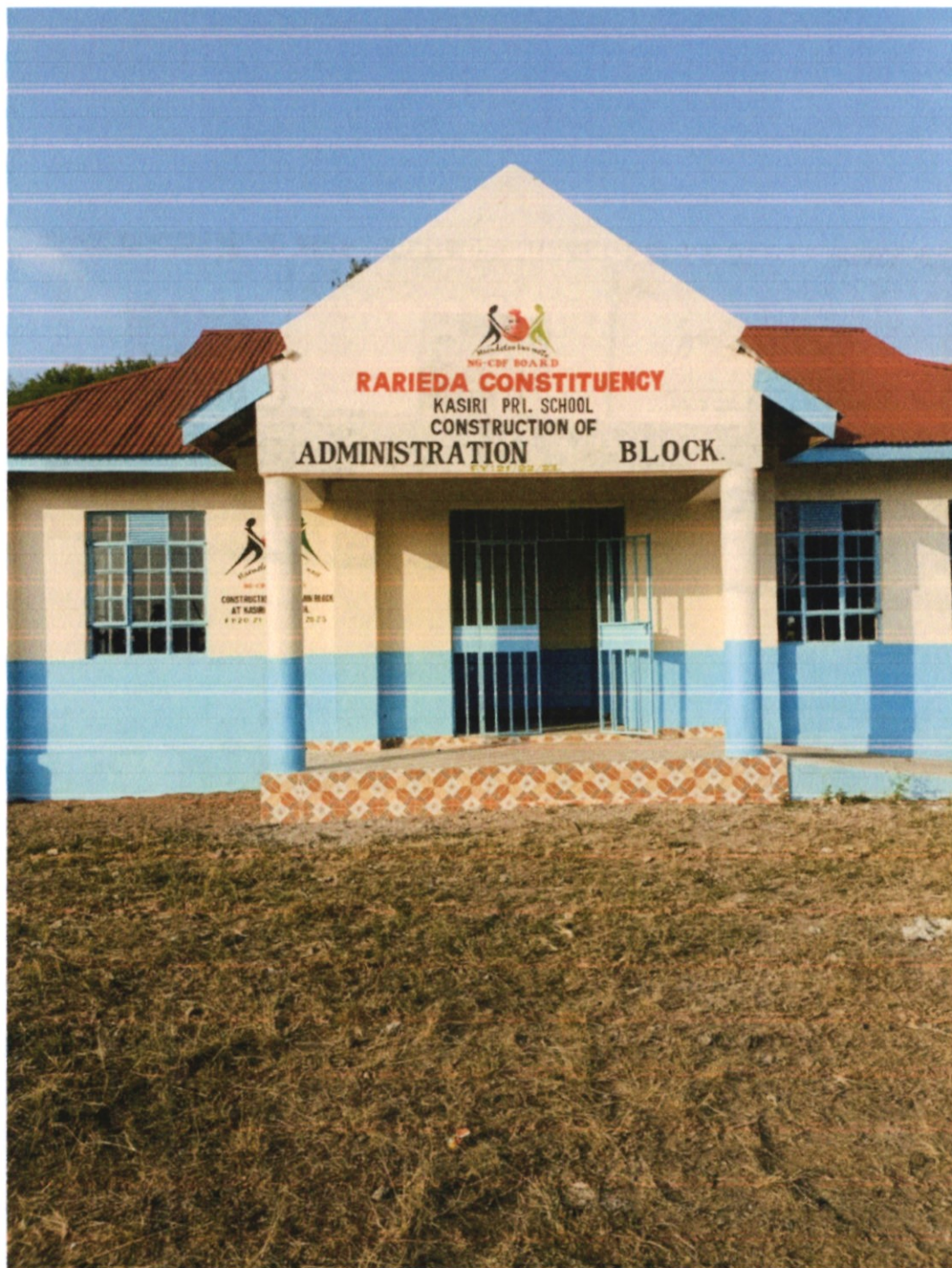
Figure 7: Administration Block at Kasiri Primary School
