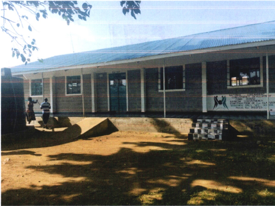
Figure 15: Construction of 1No. Classroom at Nyakongo Girls secondary School
