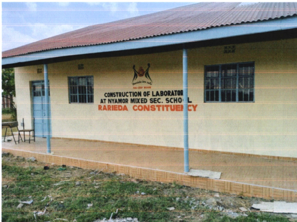
Figure 7: Construction of Laboratory at Nyamor Mixed Secondary School
