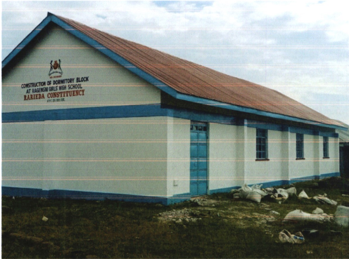
Figure 9: Construction of Girls Dormitory at Ragengni Girls secondary school
