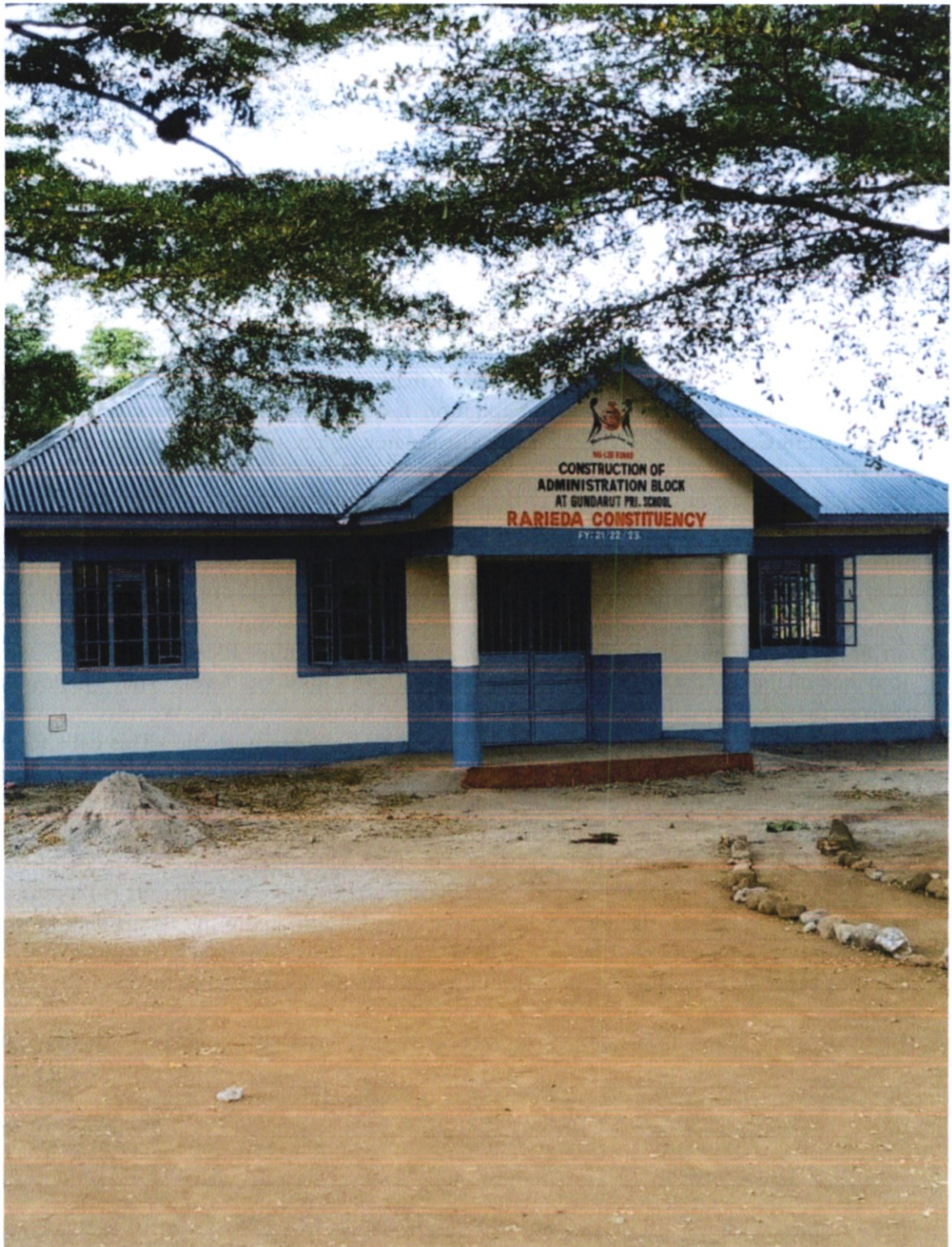
Figure 1: Gundarut Primary School, Completion of Administration Block, Front View.
