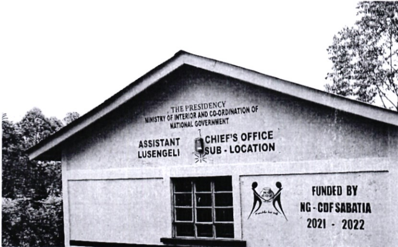
Complete construction of Lusengeli Assistant chief's office
