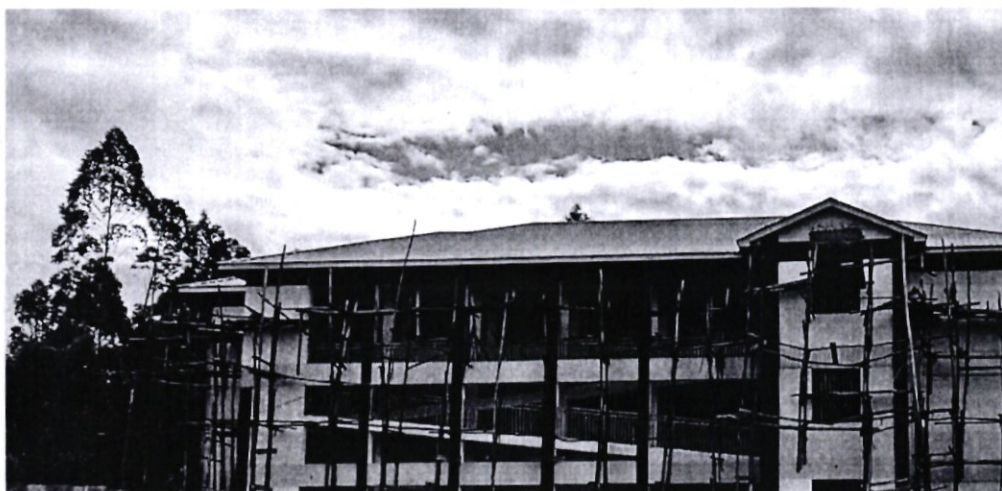
Image 3: On-going construction at KMTTC – Vihiga
