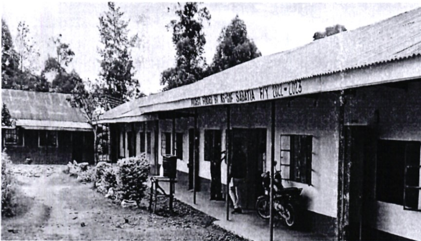
Complete Renovation 3 No. classrooms at Mulundu Primary School.
