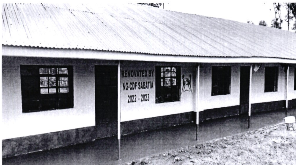
Image 4: Complete Renovation of Classroom at Mudete Primary
