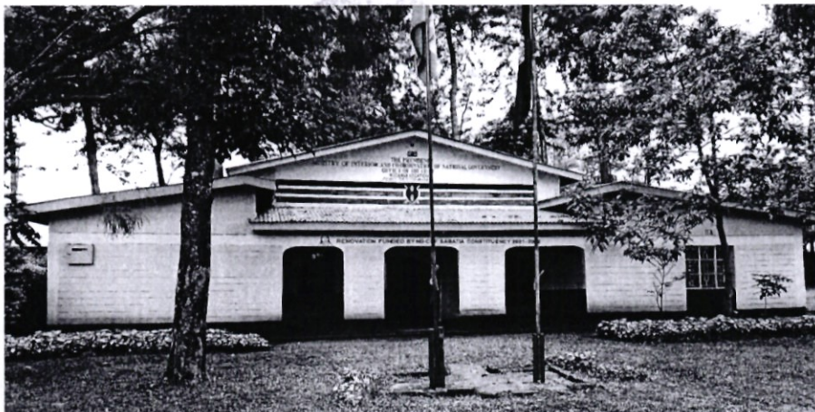
Image 2: Complete Renovation of Wodanga Chief 's office
