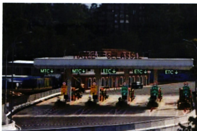
The Haile Selassie CBD exit completed in December 2023 had recorded over 800,000 vehicle exits by end of June 2024.
